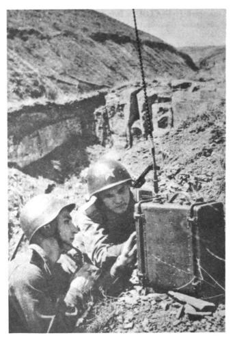
Figure 6-64. Field radio equipment. Soviet tactical radio sets are generally rugged and reliable, but somewhat heavy in weight.
